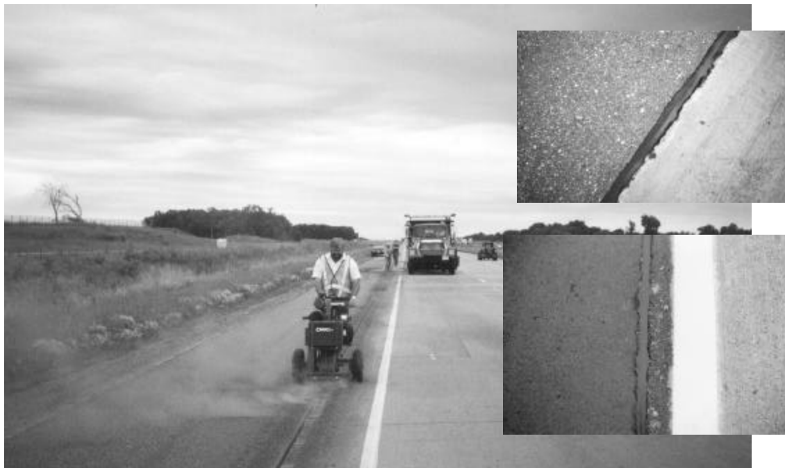
Figure 6: Route and Seal according to Mn/DOT Specification
