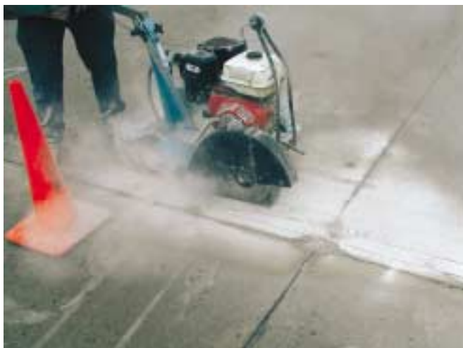
A failed joint is sawed in preparation for replacement.
