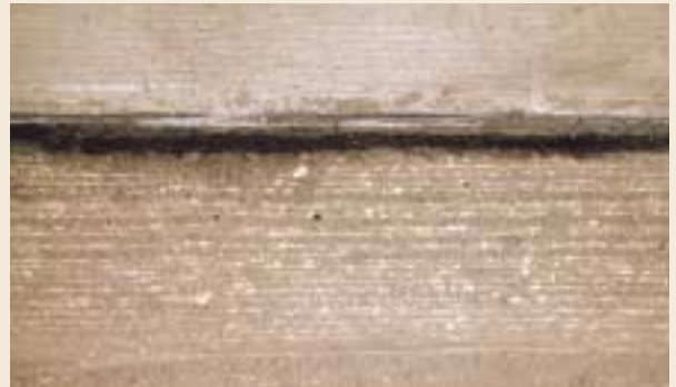
Grinding is used to prepare a longitudinal joint for repair.
