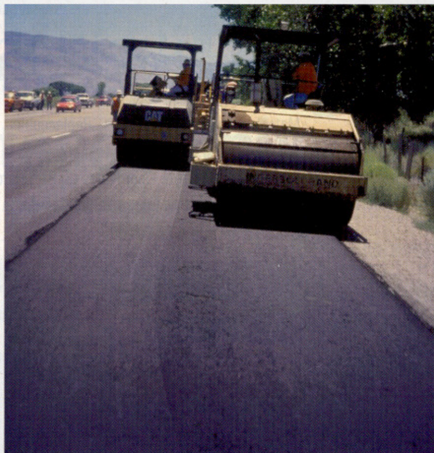
For most asphalt concrete mixtures that exhibit tender characteristics, the tender mix must be compacted to as high a density as feasible, as quickly as possible. For most tender HMA mixtures, that means placing two rollers on the mat within the upper temperature zone.
