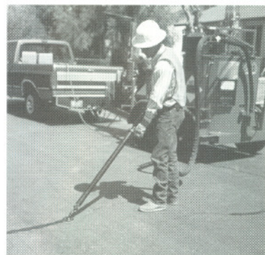
Crack sealing is a first line of defense in pavement preservation.
