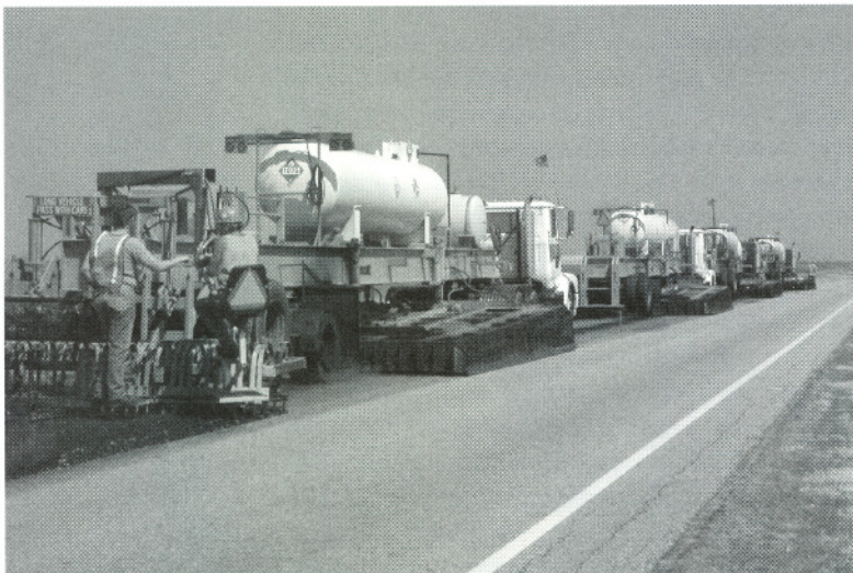
Hot in-place recycling asphalt train replacing roadway surface in one pass.
