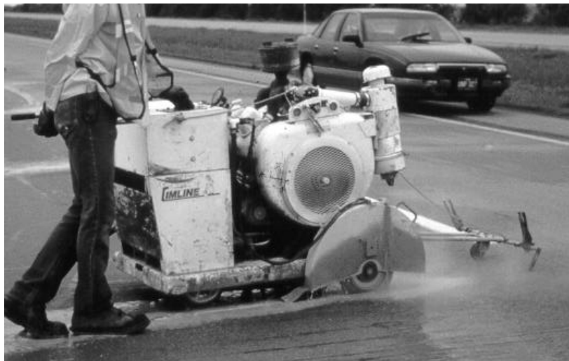
Figure 7. Concrete joint saw.
