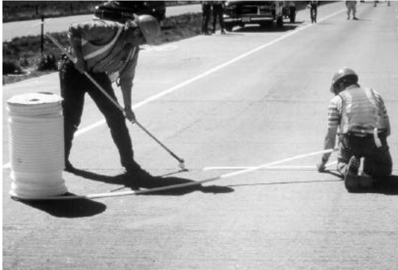
Figure 16. Backer rod installation.
