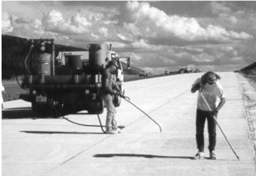
Figure 18. Silicone sealant installation.
