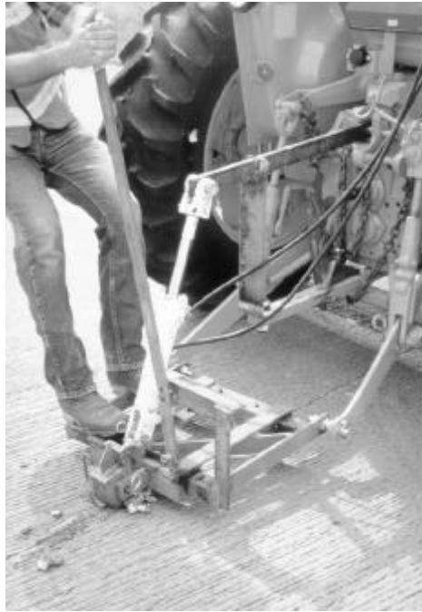
Figure 12. Joint plowing operation.
