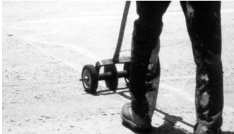
Figure 10. Hand-operated backer rod installation tool.
