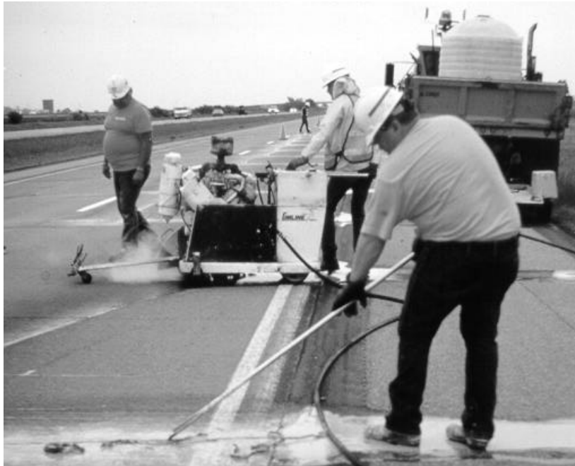
Figure 13. Joint resawing operation.
