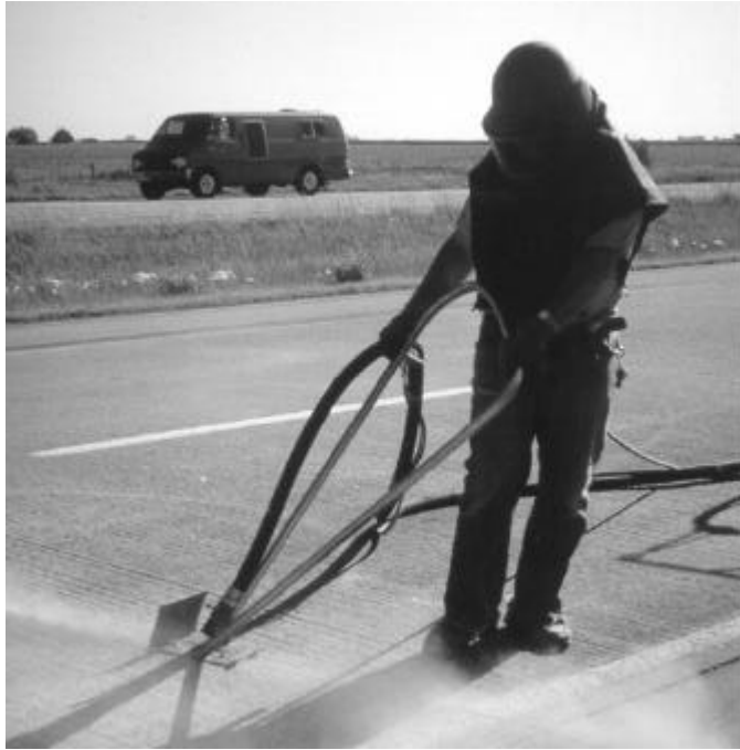
Figure 14. Abrasive blasting operation.
