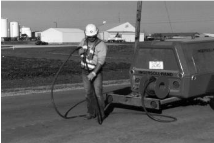
Figure 9. Airblasting operation.
